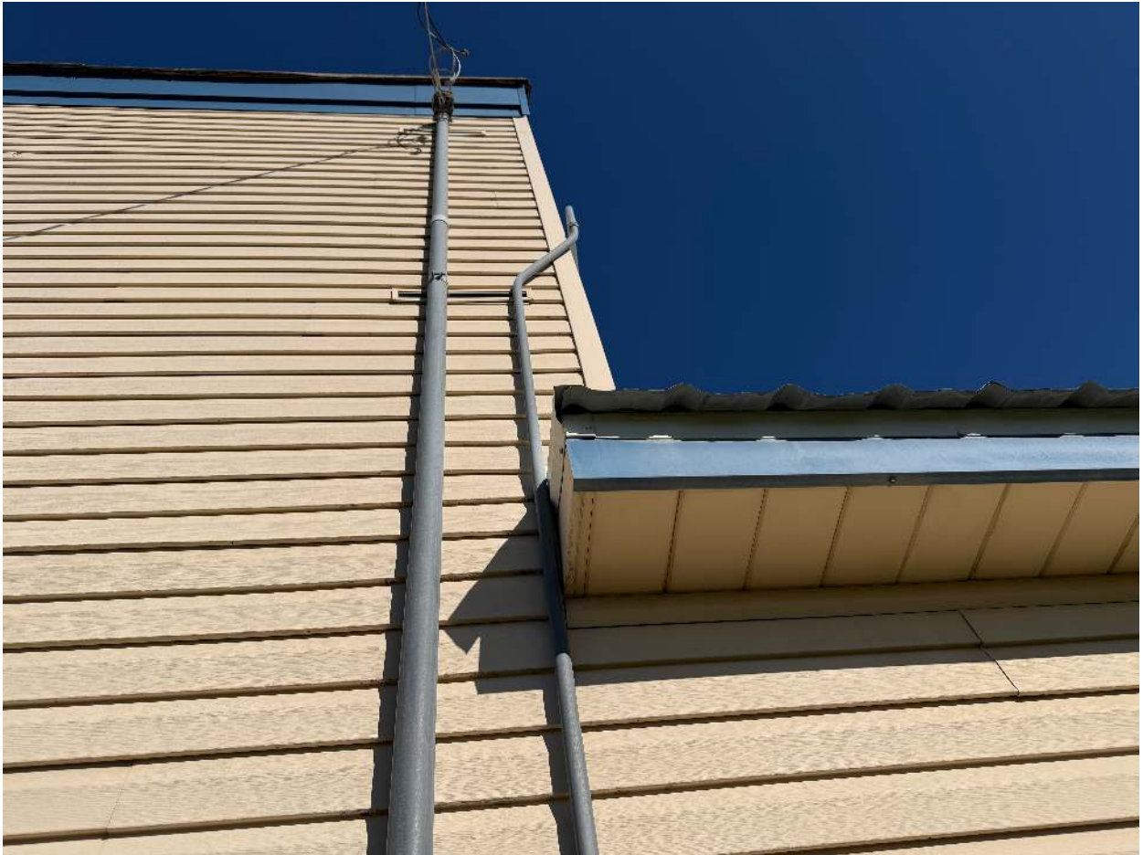
Detail showing the junction of the main arched volume and lower attached section.
