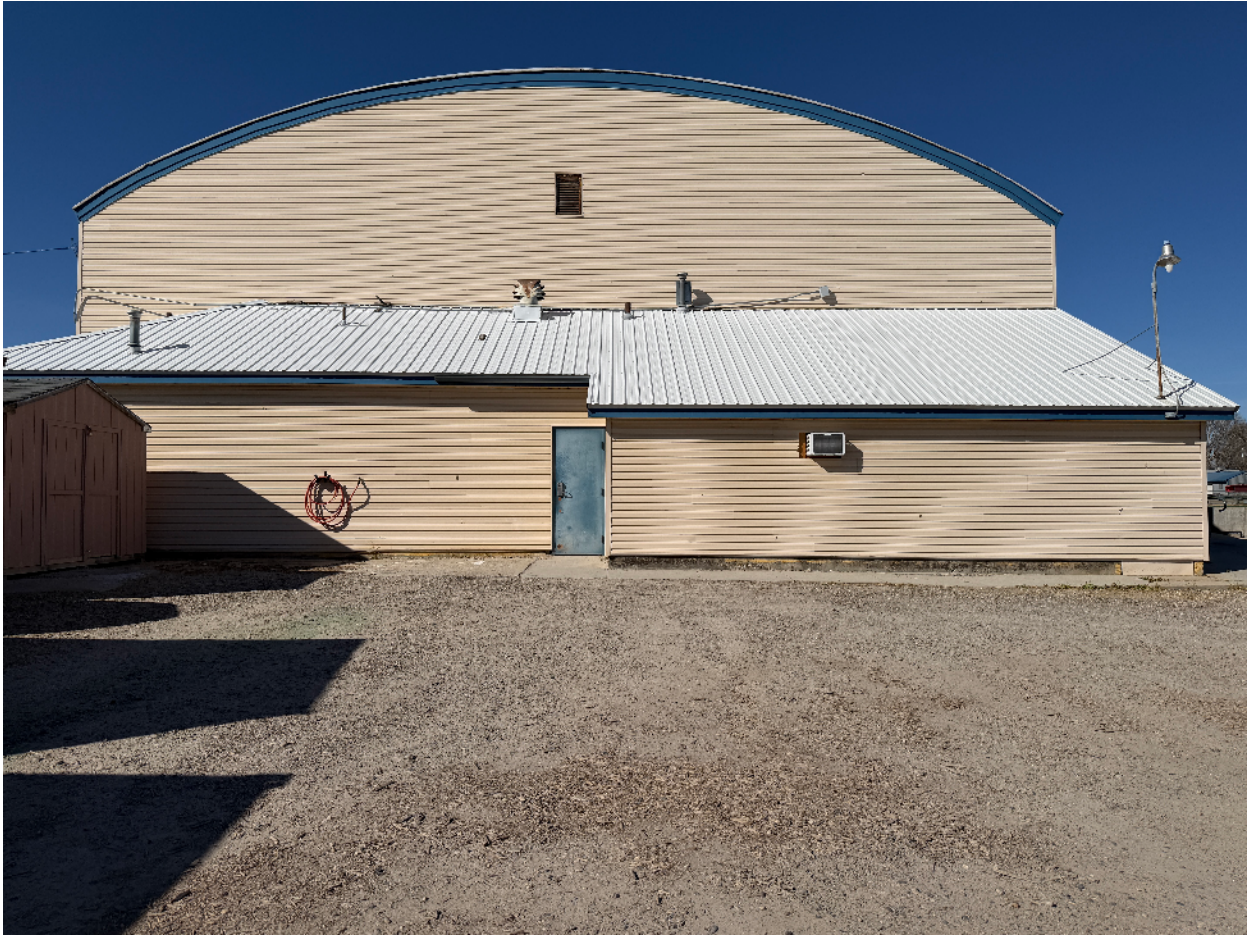
Nearly direct end view showing the arched wall profile and lower attached section.
