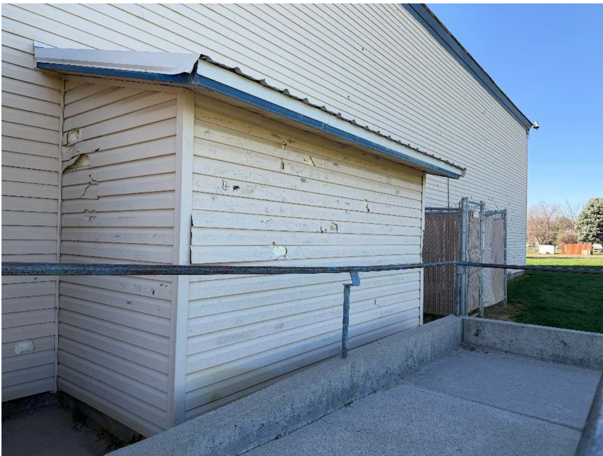
View showing the side and rear of the lower entrance section and accessible ramp construction.
