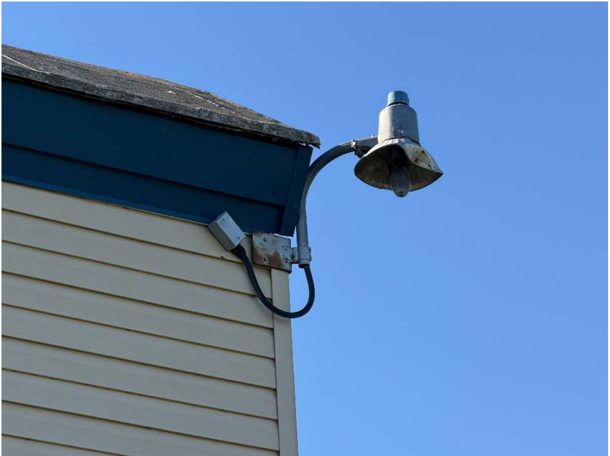
Detail of an exterior light fixture and the roof-edge treatment.
