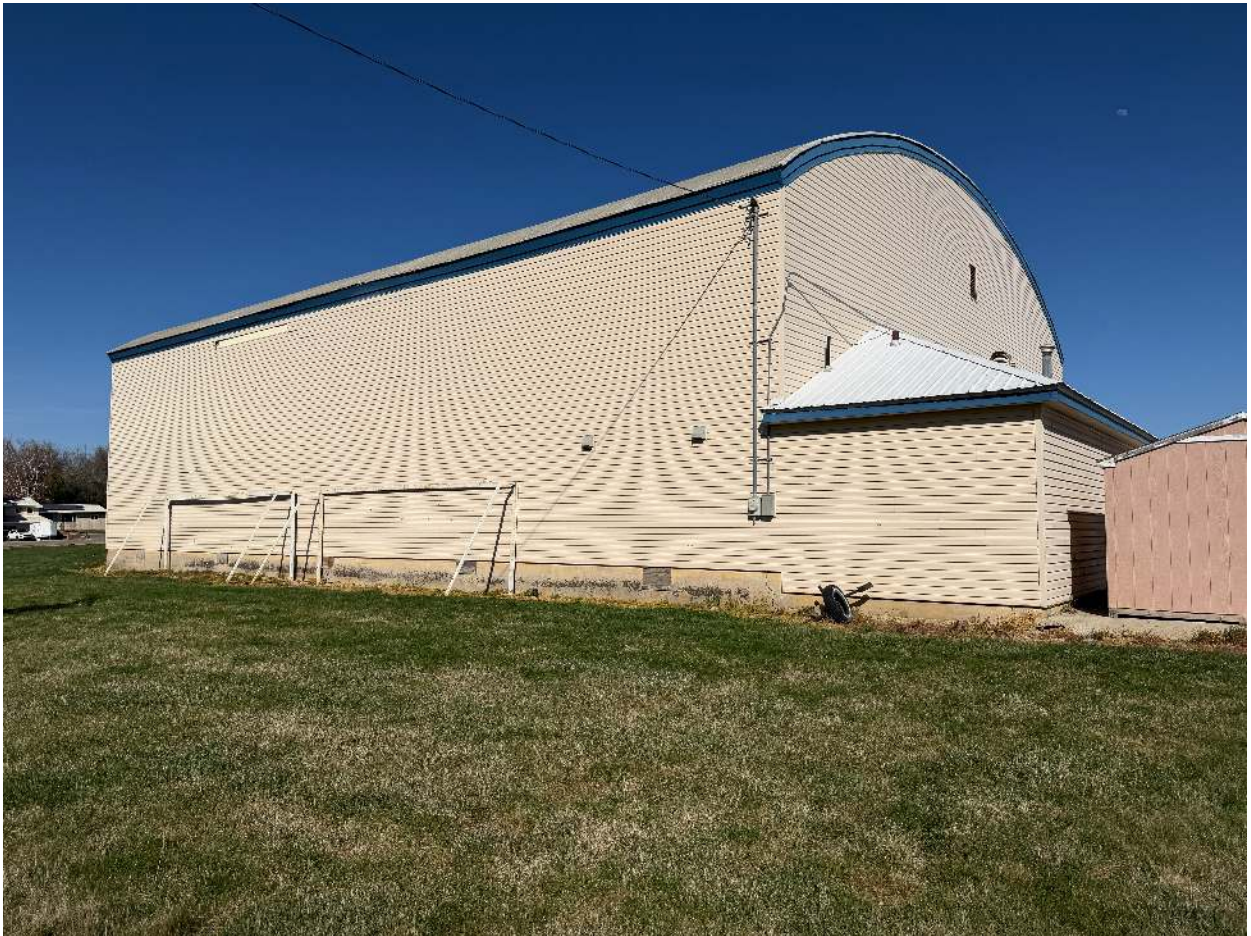
Oblique view showing the long wall, curved roof profile, and lower attached section.
