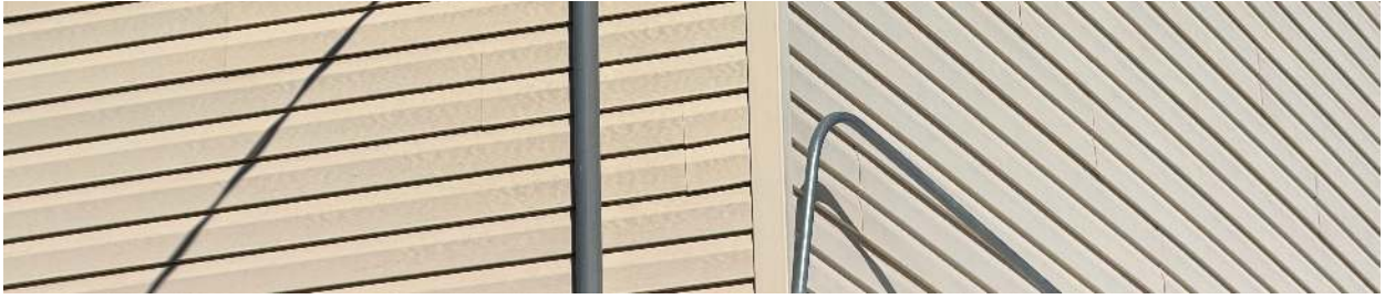
Detail of the curved roof edge, horizontal siding, trim, and exterior utility installation.
