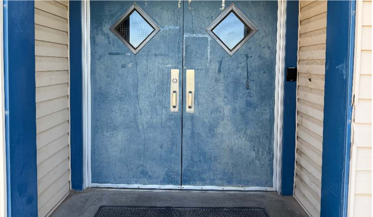
Detail of the double-leaf entrance doors with diamond-shaped lights and metal hardware.
