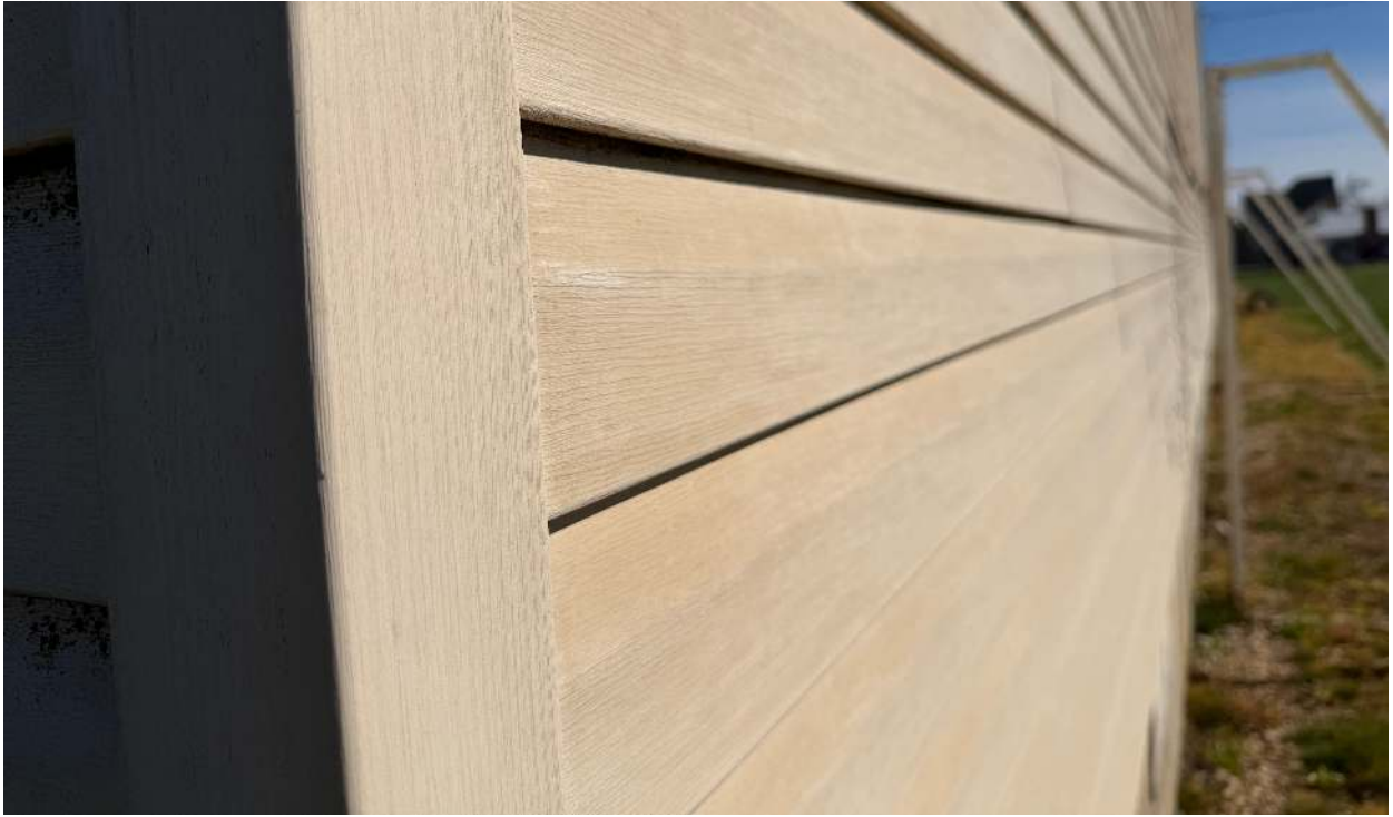
Close view documenting the horizontal wall cladding and its condition.
