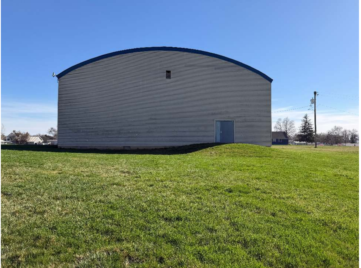
Direct end view showing the arched wall profile, small upper vent, and service door.
