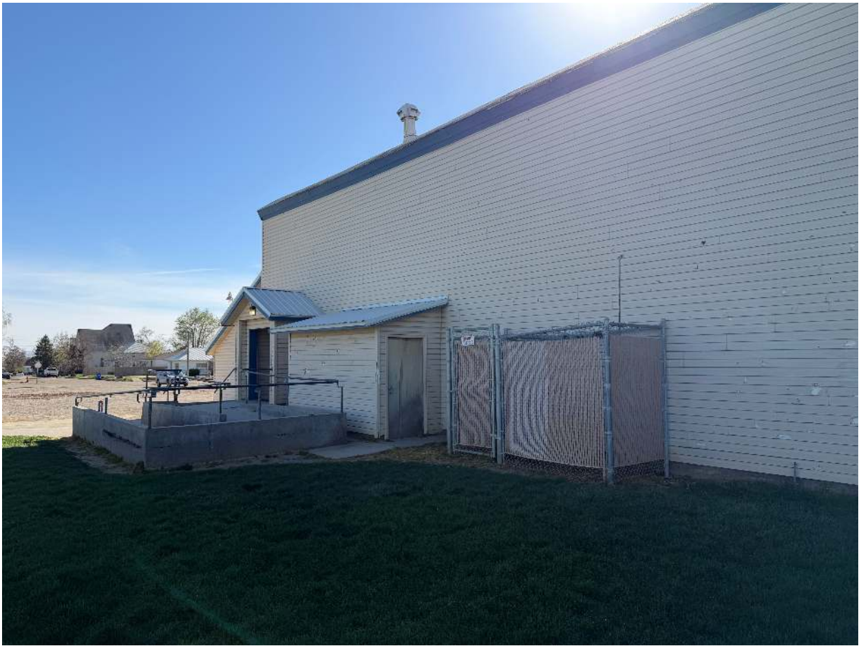
Oblique view showing the long wall, attached enclosures, accessible ramp, and principal building mass.
